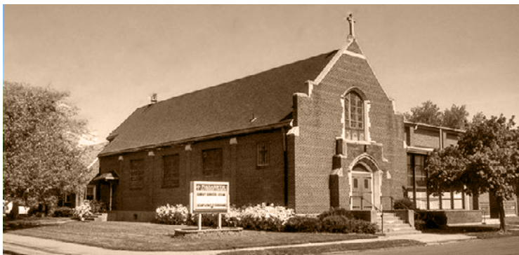
Branch members have performed ongoing maintenance around Nazareth Lutheran Church including painting and cleaning, repairs to the boiler room, upgrading the air filters to comply with CDC requirements, vacuuming and ground maintenance, snow removal, mopping the basement, and setting up and serving coffee for fellowship.
